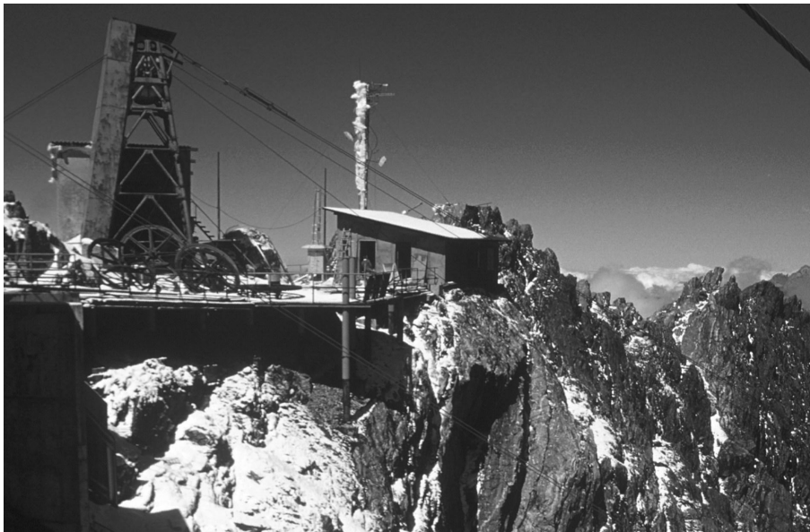
Figure 1: View over Pico Espejo with the building for the measuring instruments.
